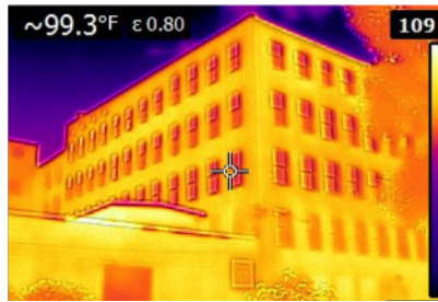
Thermal imaging of the Maryland Center for Veterans Education and Training (MCVET) in Baltimore indicates building heat gain prior to MEA-funded insulation and other upgrades.
